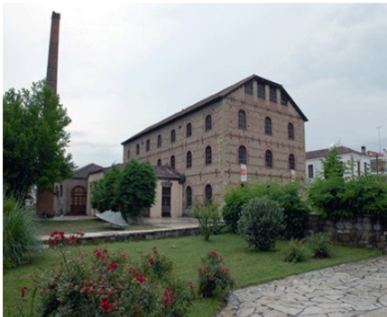
The Mill of Matsopoulos
